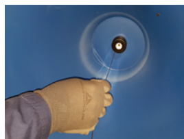
Feed the wire through the cone
